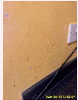
3:8 Walls Wall cleaning
