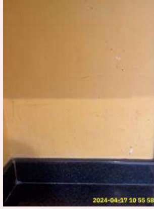
3:8 Walls Wall cleaning
