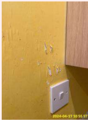
3:8 Walls Wall cleaning
