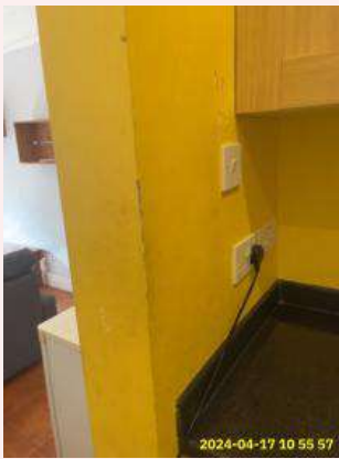
3:8 Walls Wall cleaning
