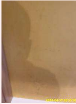
3:8 Walls Wall cleaning
