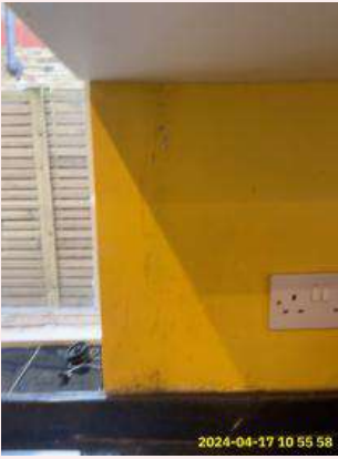
3:8 Walls Wall cleaning
