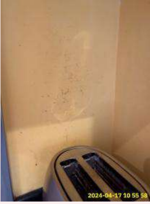
3:8 Walls Wall cleaning
