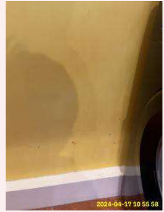
3:8 Walls Wall cleaning
