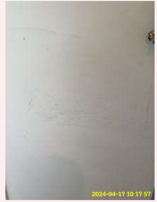
1:3 Doors Scratches on the front door
