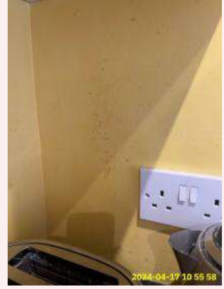
3:8 Walls Wall cleaning
