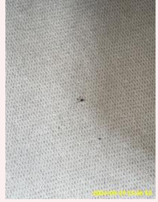
6:4 Flooring Stain - Tenant cleaning
